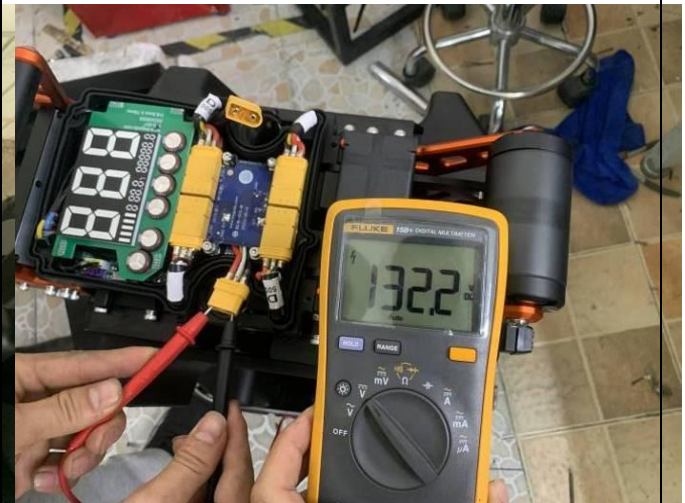
Battery voltage check
