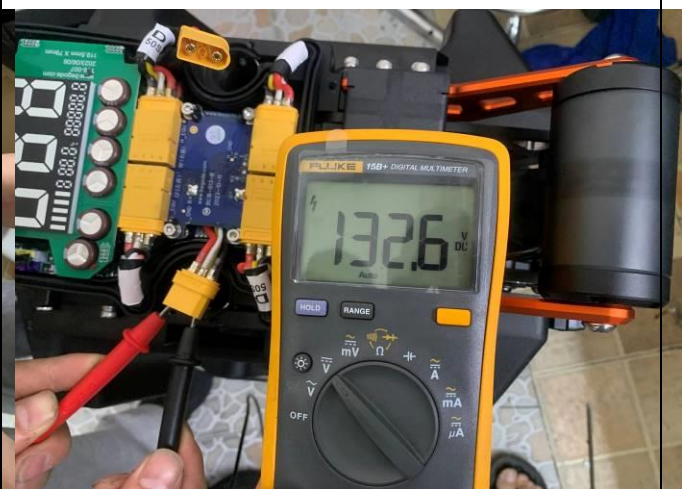
Battery voltage check
