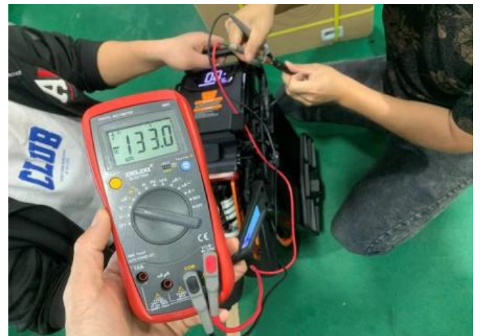
20 Battery voltage check
