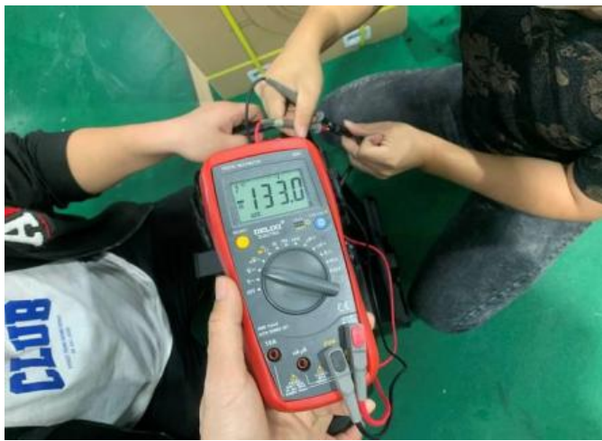
21 Battery voltage check
